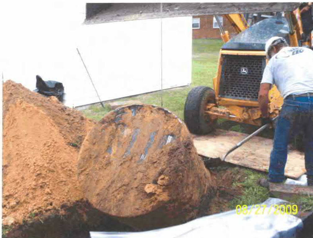
Picture 2: UST 1244Dove removal in progress.
